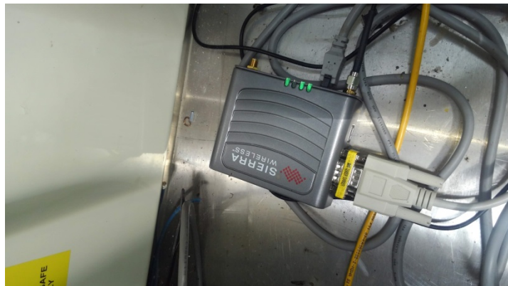
Control panel 3G modem
