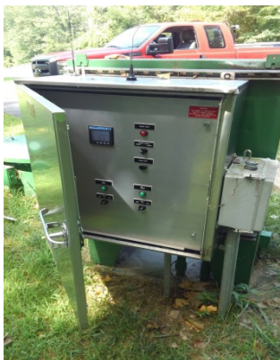
Lift station control panel
